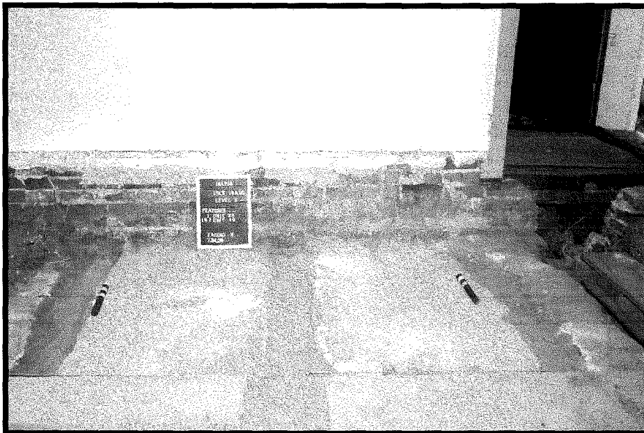
Photo Plate 10: Overview of Portions of Intact Brick Flooring (Stratum 1, Stratigraphic Unit 1), Underlying Floor Joist Trenches and Mortar Bedding (Strata 3 and 4, Stratigraphic Unit 2). Units 19 and 23, South Room, East Wing Interior.
